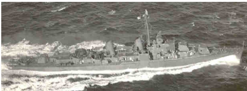
USS BARTON (DD 722) “as built” with enclosed bridge and 2 x quintuple torpedo tube mounts on 29 Dec 43 from http://www.navsource.org/archives/05/pix1/0572217.jpg
